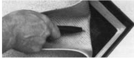
2. Make a cut from the base out to the top of the flooring in line with the mitre.
