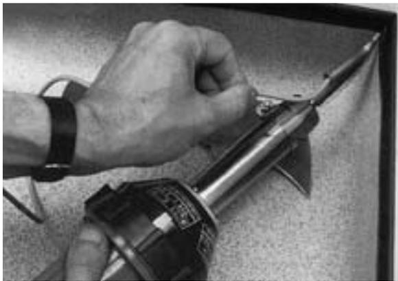
1. Groove the internal mitre before welding.
